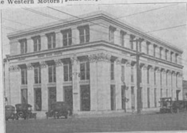
Western Motors Co., Building, at San Francisco, Cal.
